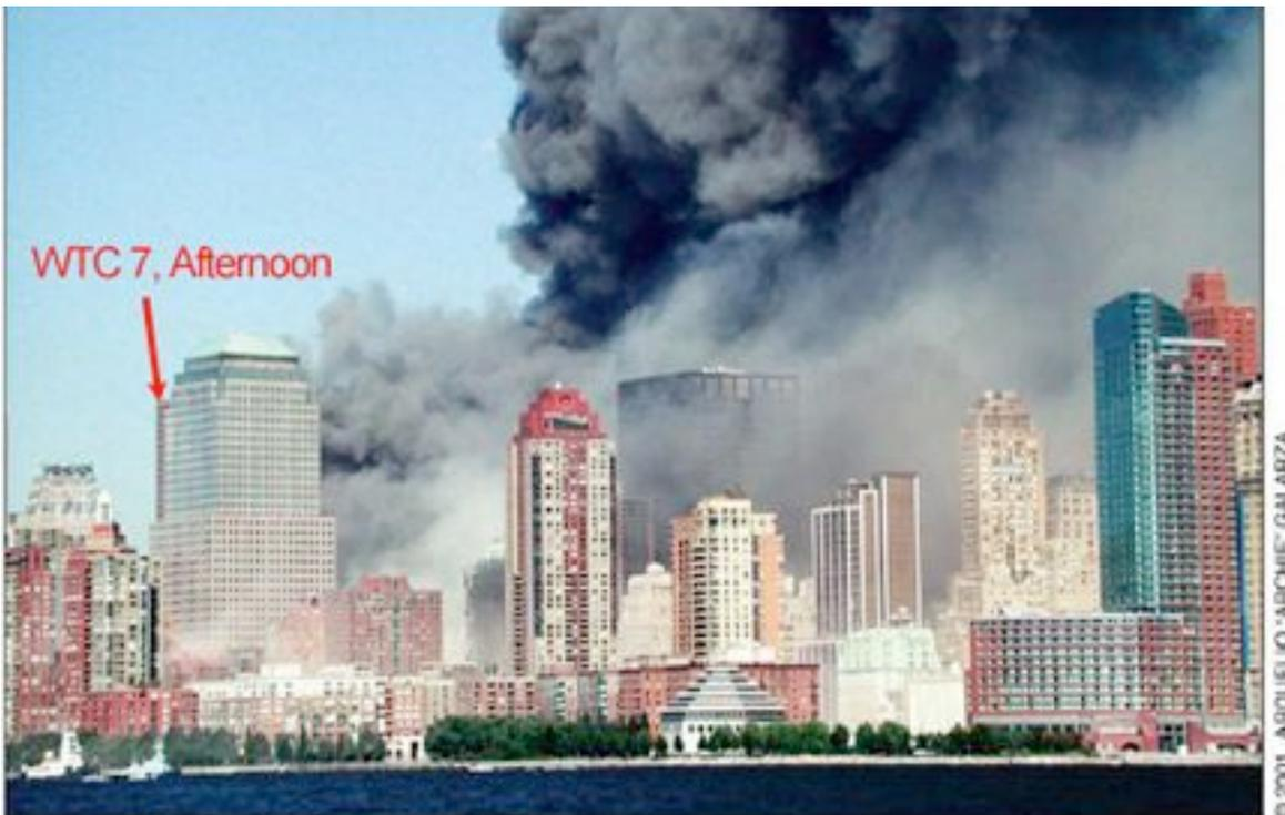
*Figure 5-18 WTC 7, with a large volume of dark smoke rising from it, just visible behind WTC 1 (left). A much smaller volume of white smoke is seen rising from the base of WTC 7. Note that the lower, lighter-colored smoke (to right) is thought to be from the two collapsed towers*
