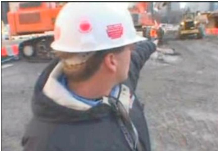
**“We’ve got the cables attached in four different locations going up. Now they’re pulling the building to the north. It’s not every day you try to pull down a eight story building with cables.”**
